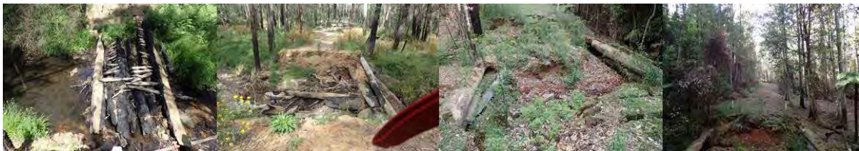
Figure 9 Burnt or destroyed bridges dramatically restricted access
